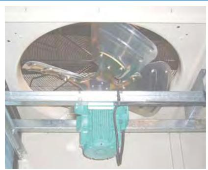
The motors are factory wired to chiller unit control panel where the motor starters are located to control the operation of these motors.
